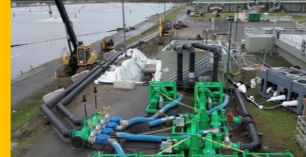
Everett, WA Wastewater Treatment
